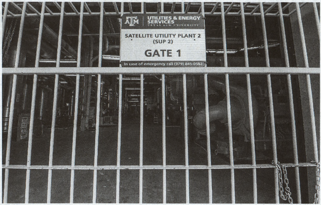
(Left) Rendering depicts the thermal energy storage tank after completion in 2016. (Right) The thermal energy storage tank will be located on West Campus near UES Satellite Utility Plant 2.
