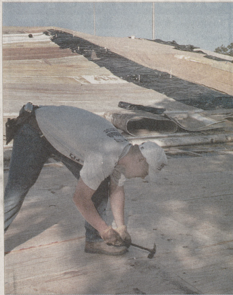
BRADLEY ATCHISON/THE BATTALION Pat Marek, a junior agricultural business major, nails down plywood Tuesday at the site of the new Mt. Aggie behind the Varsity Tennis Center.
