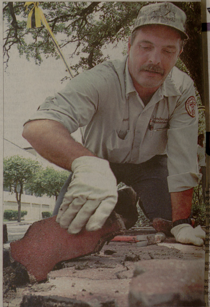
Michael Priest of Landscaping Maintenance North removes bricks from the sidewalk between the MSC and the Koldus Building Wednesday. Workers will place sand under the bricks to help level the sidewalk.
