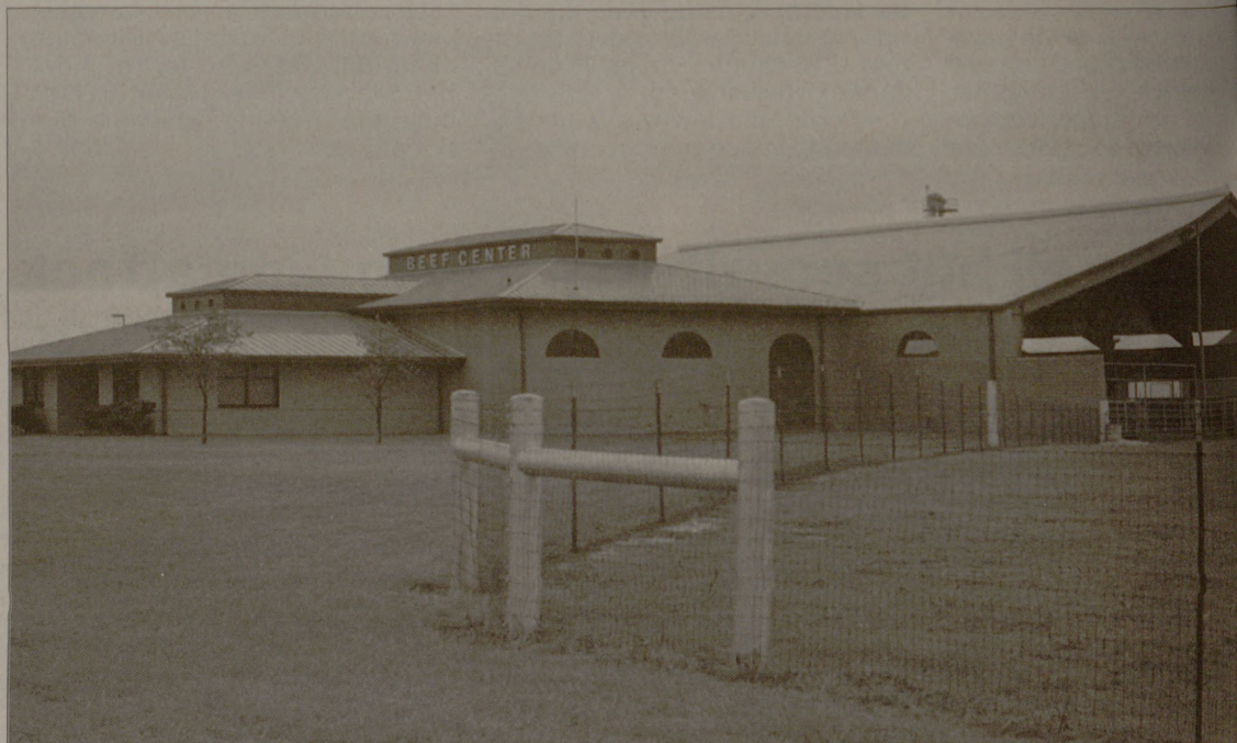
Texas A&M University's new Animal Science Teaching, Research and Extension Complex, located on Farm Road 60, will offer students expanded research and support facilities.
