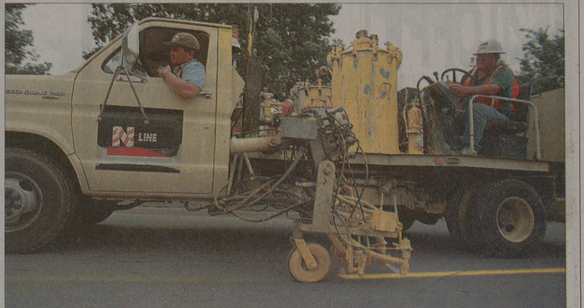
GREG MCREYNOLDS/THE BATTALION Todd England and Bob England paint two-way stripes on Welsh Street Thursday afternoon.
