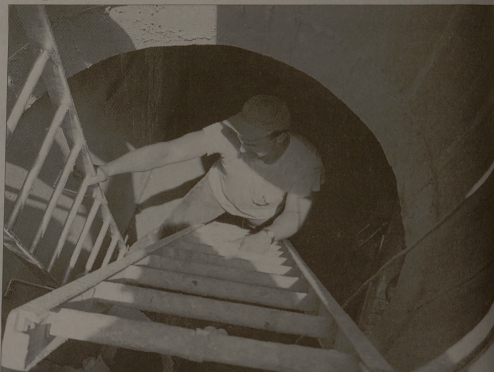
Plumber Scott Bates watches as Lee Sharp, a senior construction science major, drills holes in ladders and valve boxes to prepare the water pipes between the Central Campus Parking Garage and the new Library Extension and Computer Lab to pass safety inspection.
