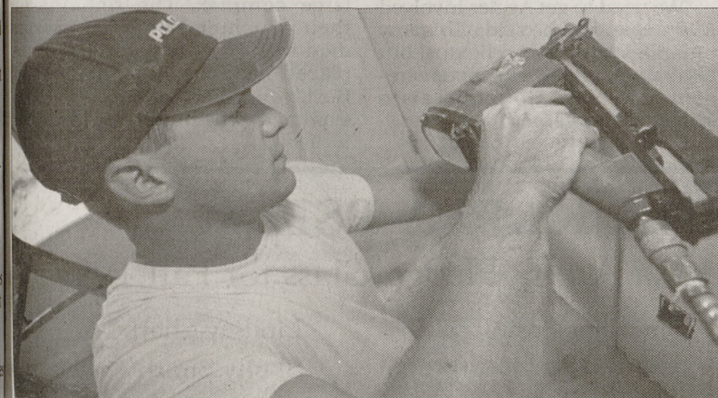
DEREK DEMERE/THE BATTALION Ryan McMahan, Class of '96, nails molding to a wall with a pneumatic nailer.
