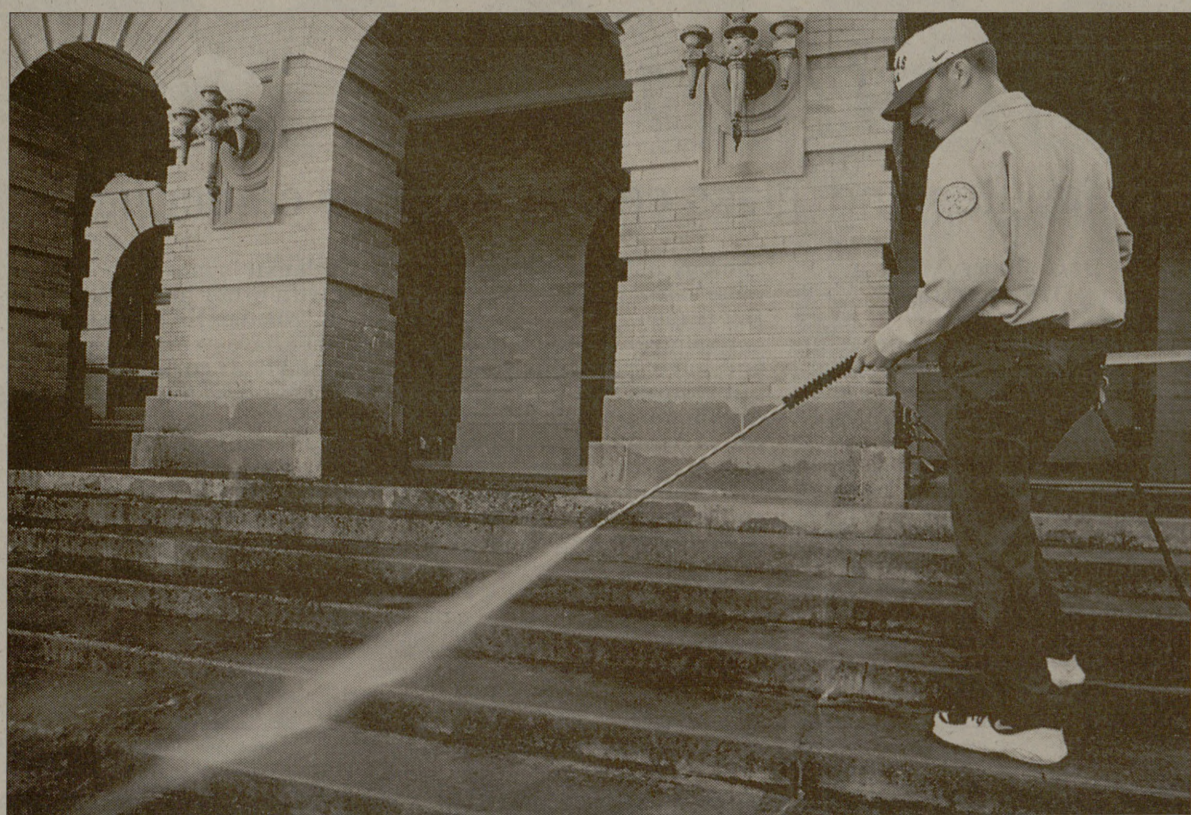
Damn birds! Chad Lippey, a maintenance worker for area 3, is power washing the steps of the Academic Building. Dave House, THE BATTALION
