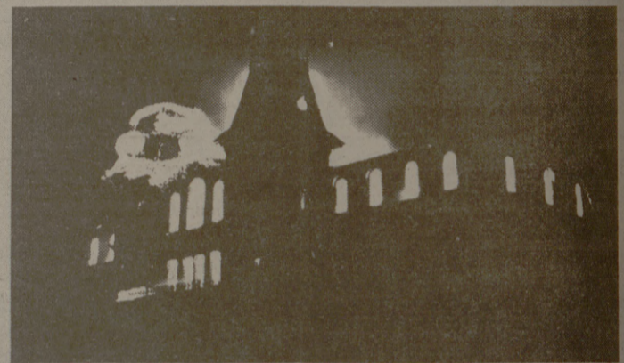
The cause of the Old Main fire has never been determined.
