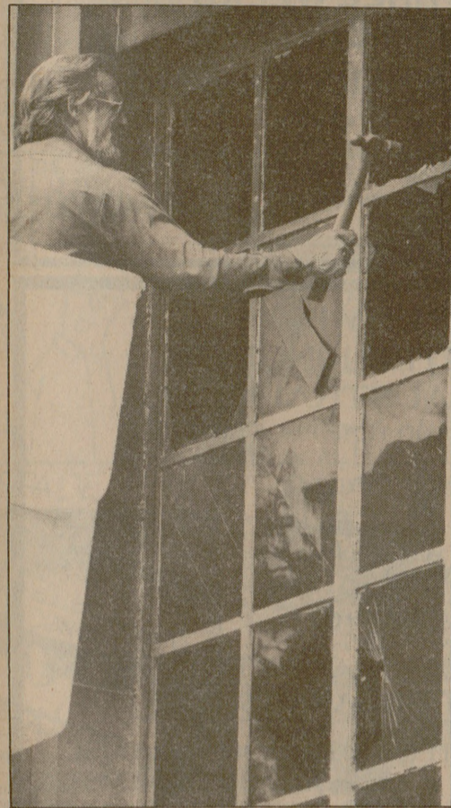
Physical plant employees knock out the remaining glass of windows in the Chemistry Building after the explosion Tuesday. After sweeping up the glass, the men boarded up the windows, leaving one open until water in the lab room dries out.
