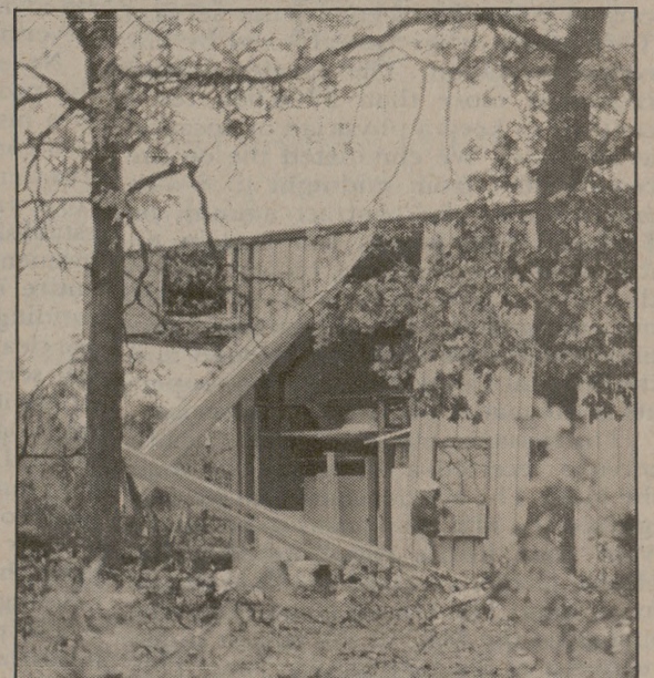
This is one of many buildings hit by tornadoes.
