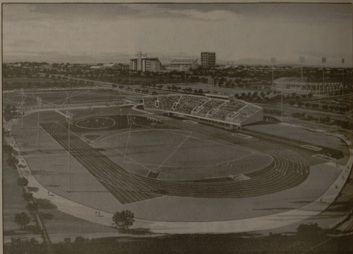
Phase I of the Frank G. Anderson Track and Field Complex (above) is scheduled to be completed March 8 in time for the A&M track teams to host their first meet in over three years.
