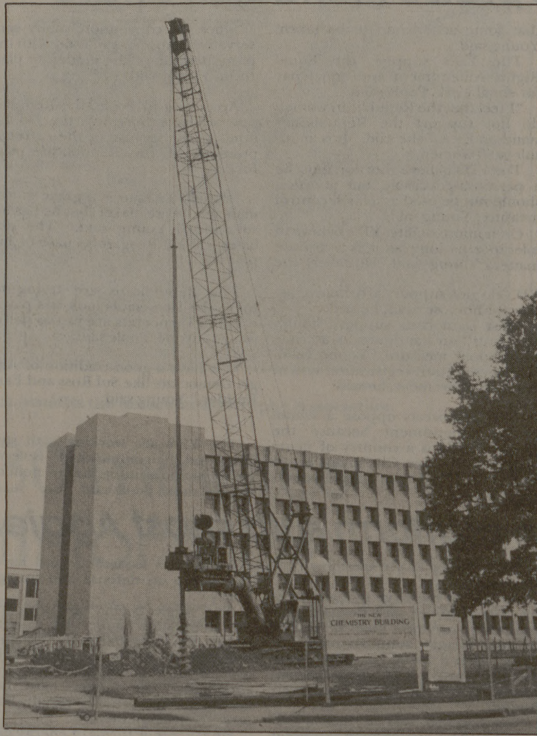
Construction of new chemistry building.
