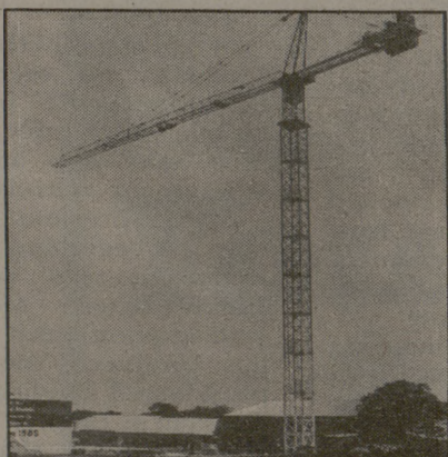
Construction on the new Hilton continues.
