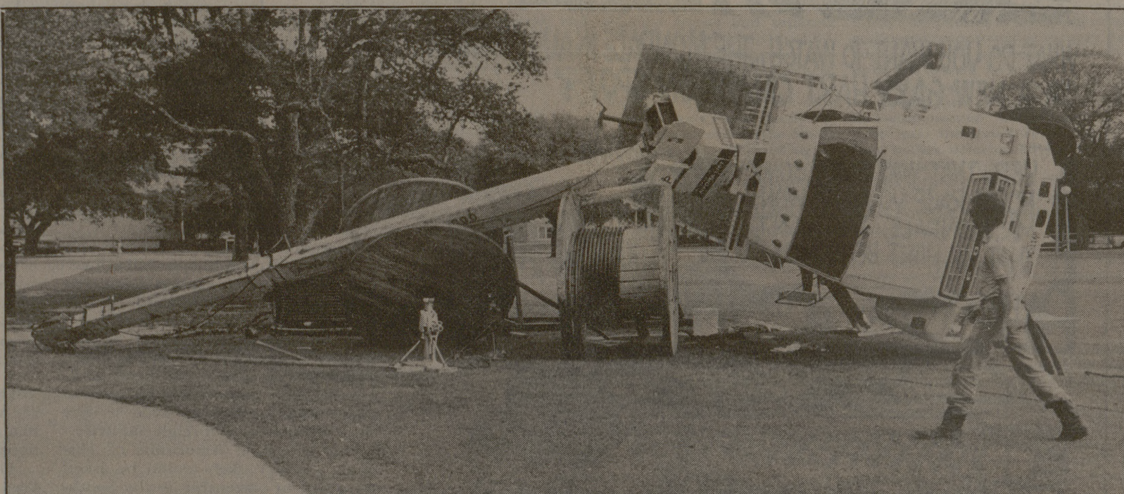
Fallen crane truck
