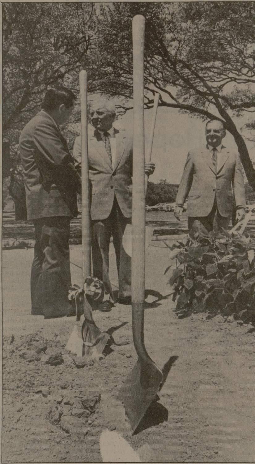
Ford D. Albritton (center) is congratulated by William A. McKenzie as Royce E. Wisenbaker looks on, following the ground breaking for the new bell tower at the west campus entrance.
