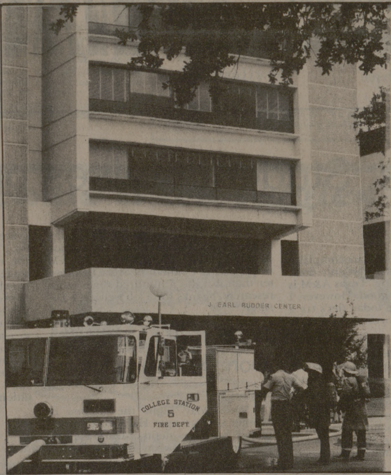
College Station firemen radio in after the Rudder Tower fire.
