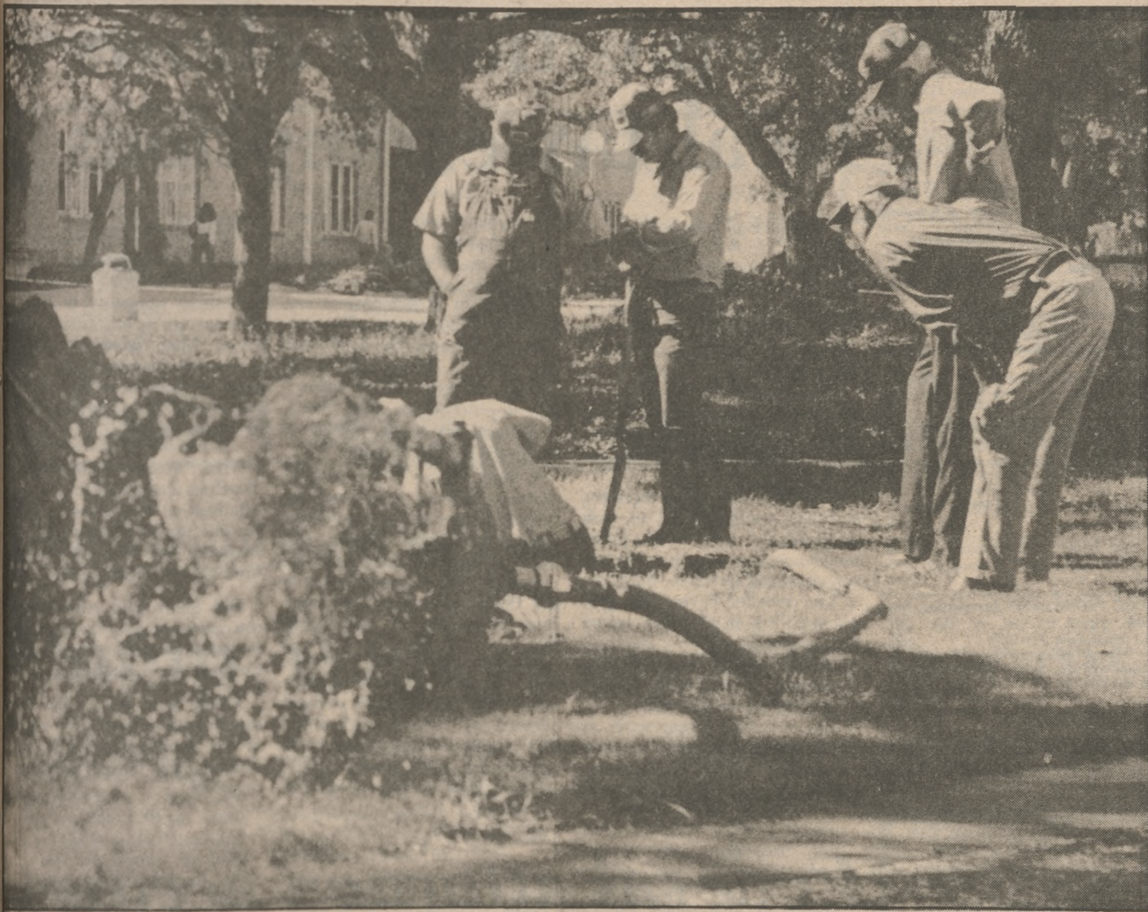
Working in the hole
