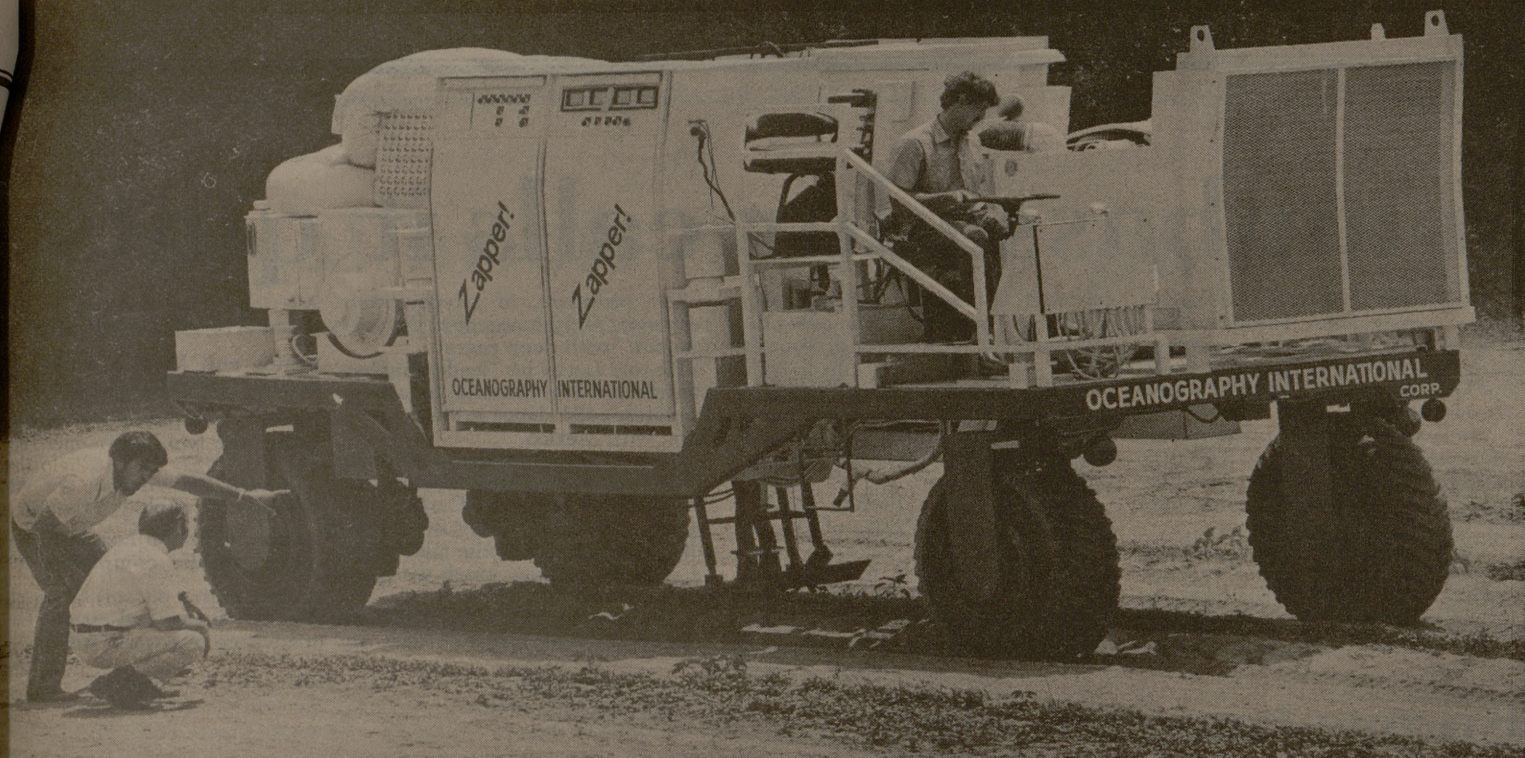
Gary Drake drives the Zapper III as Frank Davis and John Hughey watch. The Zapper III, invented by Oceanography International Corp., uses high frequency waves similar to those in a microwave oven to kill weeds in the soil.
