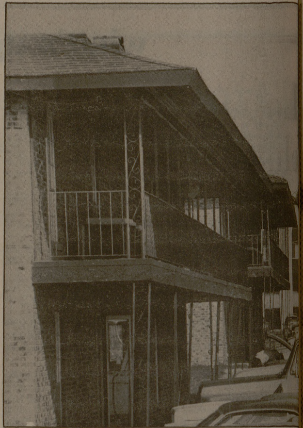
Unlike last year, Texas A&M students have been able to live in the apartments in the Bryan-College Station area this year. About 200 students found construction on their apartments unfinished when the fall semester began in 1978, but no problems have arisen this year. Battalion photo by Sam Stone.
