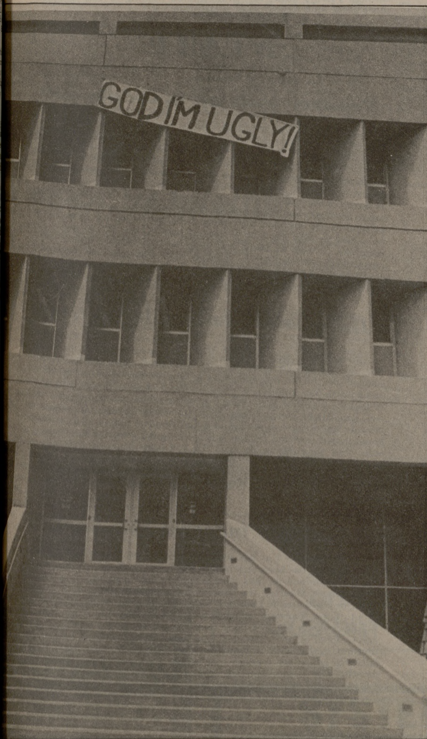
This sign on the Langford Architecture Center, hung in the fall of 1977, voiced an opinion about the building. A year later, other students, graduate students and faculty are complaining about the building — from inadequate air-conditioning to not enough privacy. Today's article is the first of a two-part series. The second half will appear in Thursday's Battalion.
