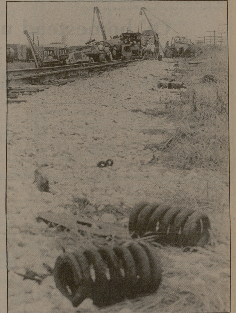
Broken remnants of railroad car wheels are scattered along the railroad tracks north of the Texas A&M campus where cars from a Southern Pacific freight train derailed last week. Here Southern Pacific work to remove one of the last derailed cars from the scene of that derailment.
