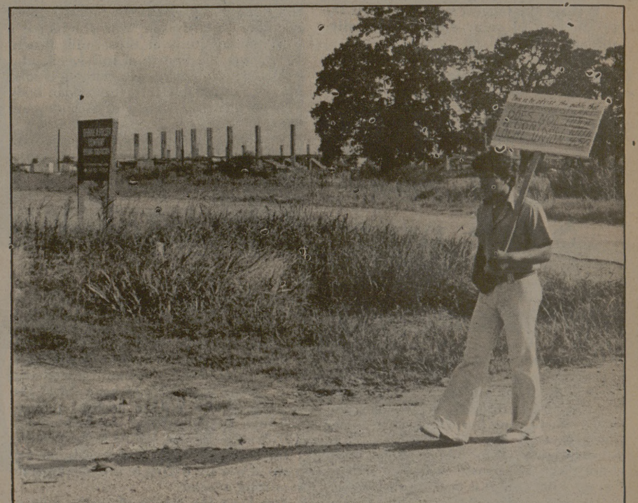
Joe Cortes, a member of Local Union 450, at the construction site of the new Texas A&M baseball field.
