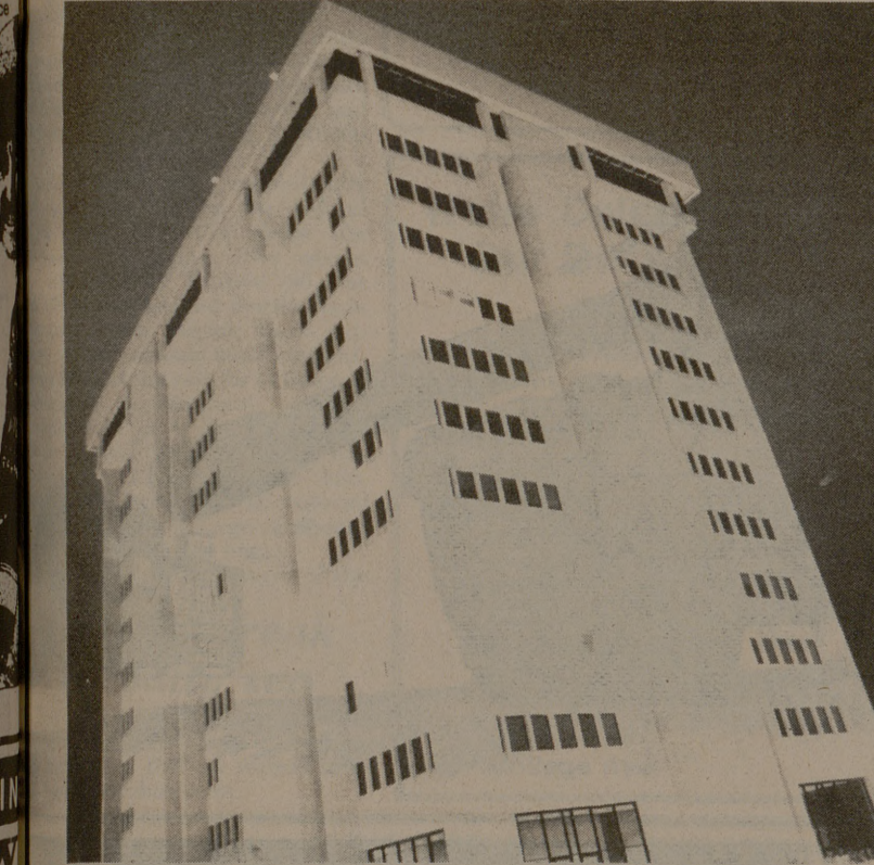
Appearances can be deceiving. Although the Oceanography Building appears to be leaning through the eyes of this photographer, building engineers insist it is perfectly straight.
