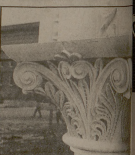
DETAIL OF COLUMN AT FERMIER HALL
