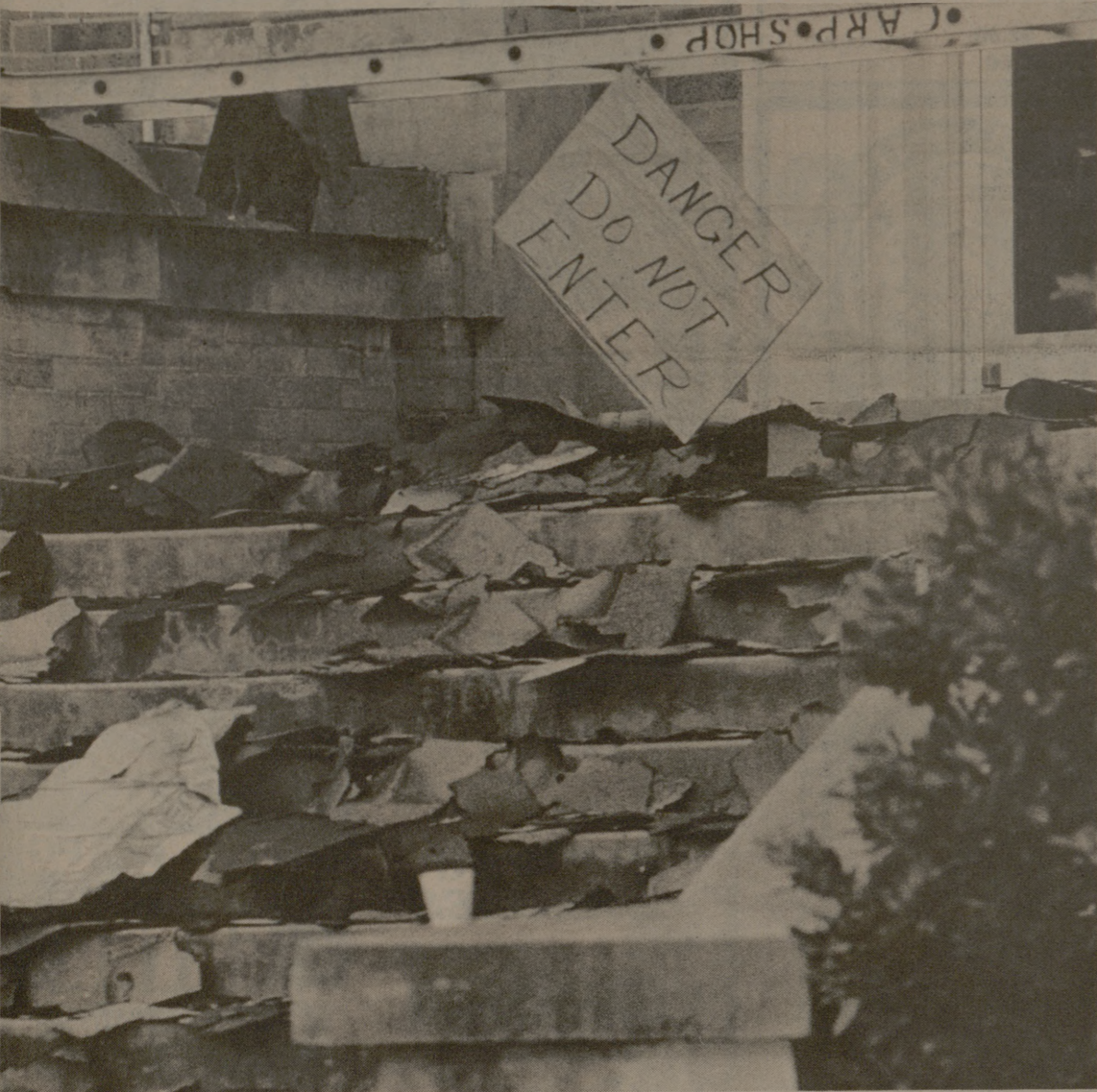
Goodwin loses leaks
