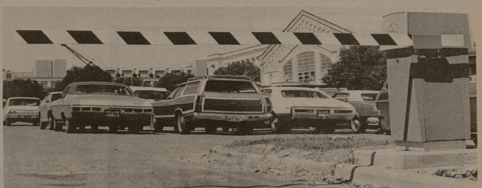
Parking gates installed
