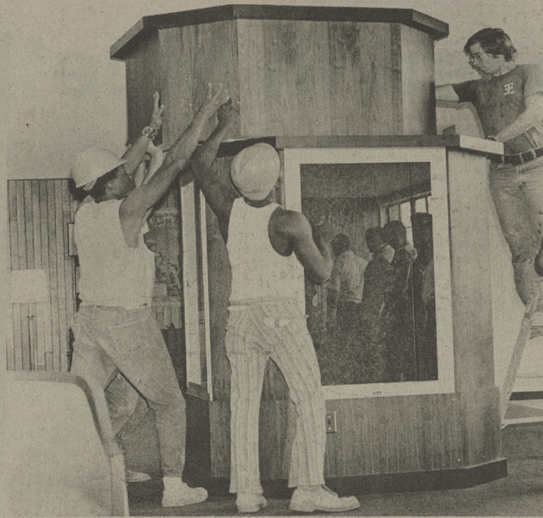
Display kiosks installed
