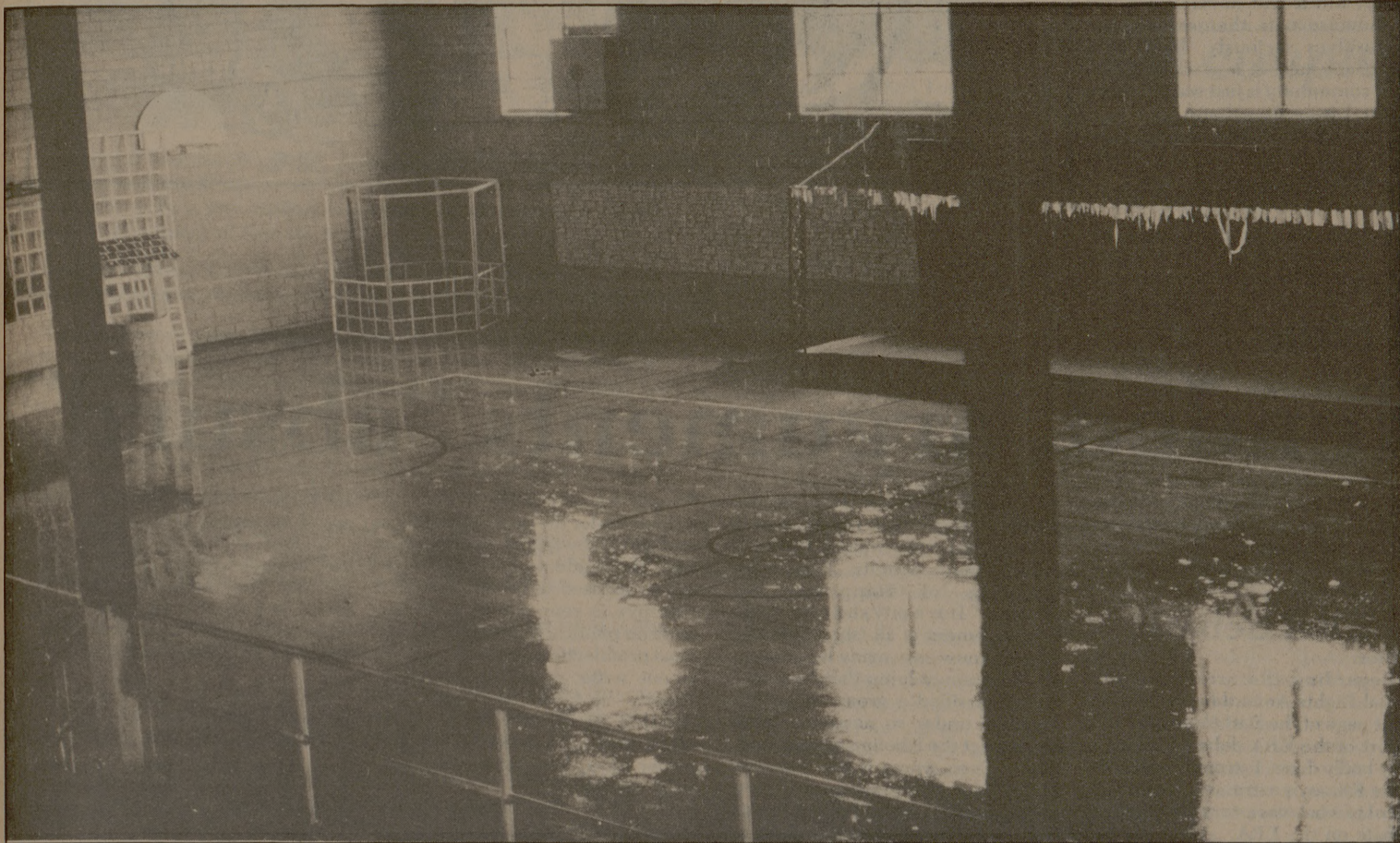
The new wooden floor of the high school gym was flooded by the rain following the high winds of the tornado. School officials called it a total loss. One
