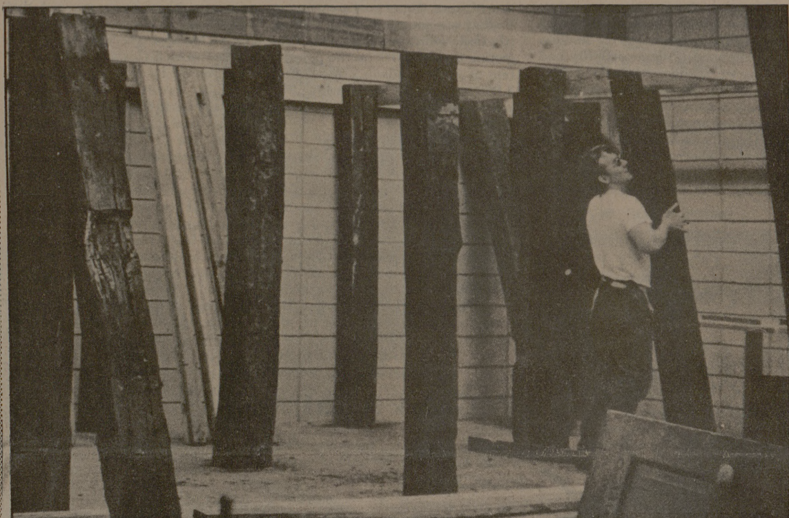
Basement gets addition
