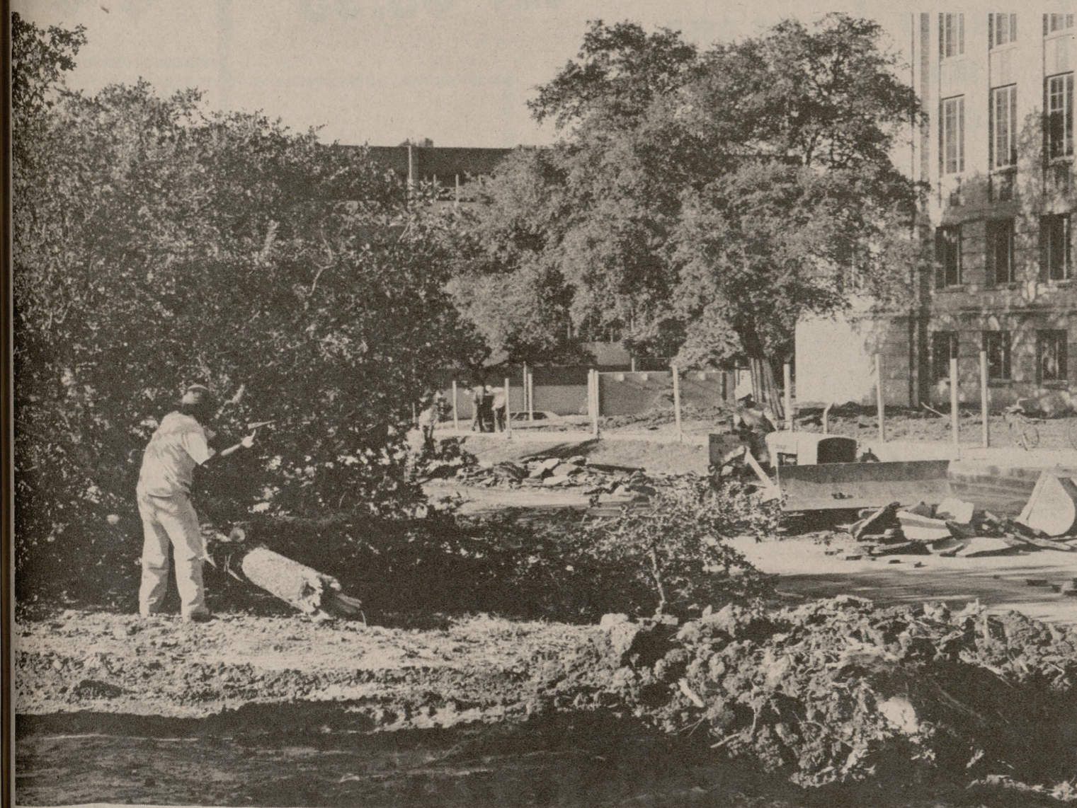
Mall construction gets underway
