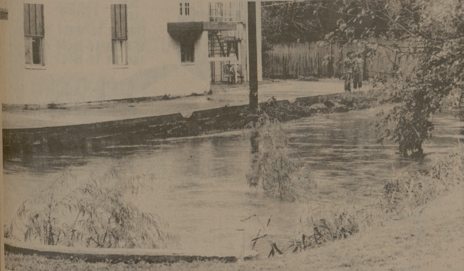
WOLF PEN CREEK again threatened to flood the Monaco Apartments in Monday's heavy rains. The flood which occurred last September rose to within a foot of the bottom of the first floor windows. (Photo by Steve Krauss)
