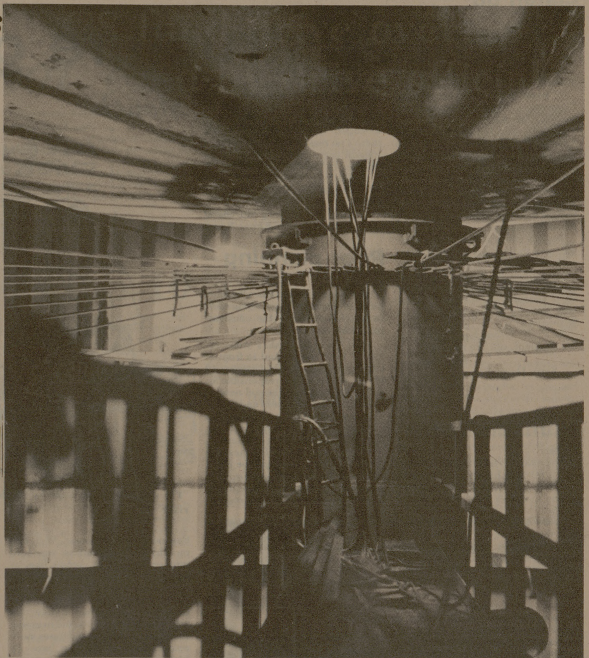
INSIDE THE TOWER presents an unusual view of the new A&M watertower. This was taken at the base of the water section of the tower which is where the tower begins to flare. (Photo by Douglas Winship)
