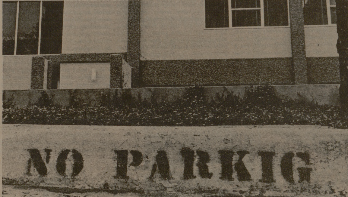
SOMETHING IS MISSING on this curbside warning in front of the Reed McDonald Services Building. (Photo by Kathy Young)
