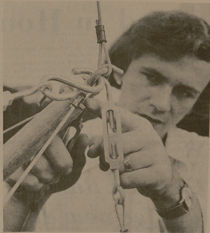
Ed Huckaby points out one of the "joints" fundamental to the stability of the tensegrity he and two other students built. (Photo by Roger Mallison)
