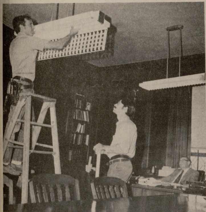
SAVING WATTS—TAMU President Jack K. Williams watches as Physical Plant Department workmen remove fluorescent tubes from his office light fixtures as part of a campus-wide campaign to reduce energy consumption. Doing the dimming are Charles Kuder (on ladder) and Ray Rowe.
