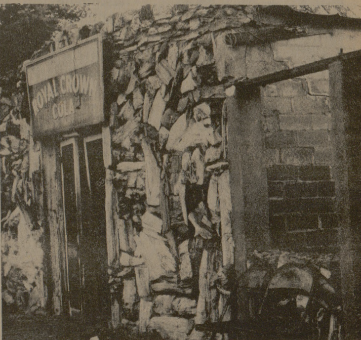
SUB-STANDARD FACILITIES typify the community of Prairie View Heights in the eastern part of College Station where CDO does most of its work. (Photo by Wayne DeVaughn)
