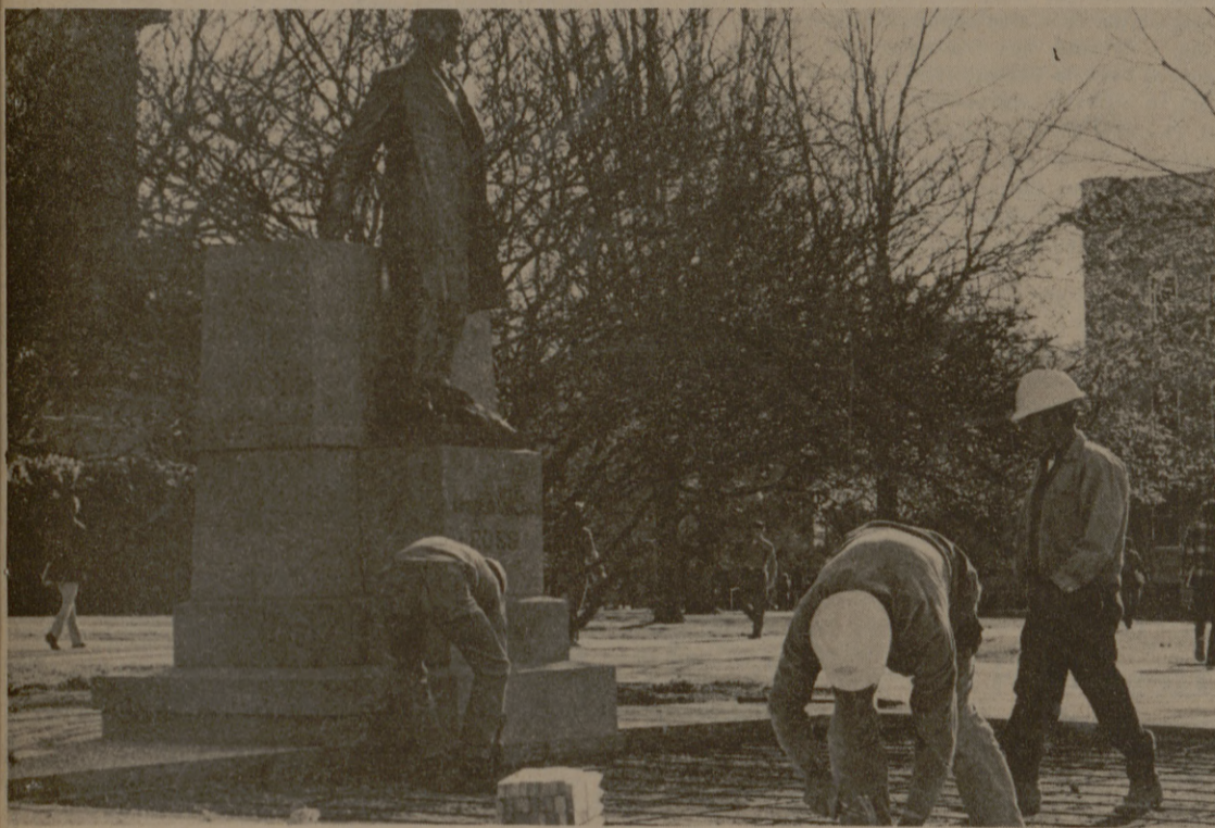
GUARDING 'SULLY' for the 1972 Aggie Bonfire took its toll on the newly installed cement in front of the statue. Workers have completed replacing the cement, which was ruined when students built fires on the surface. (Photo by Gary Baldasari)
