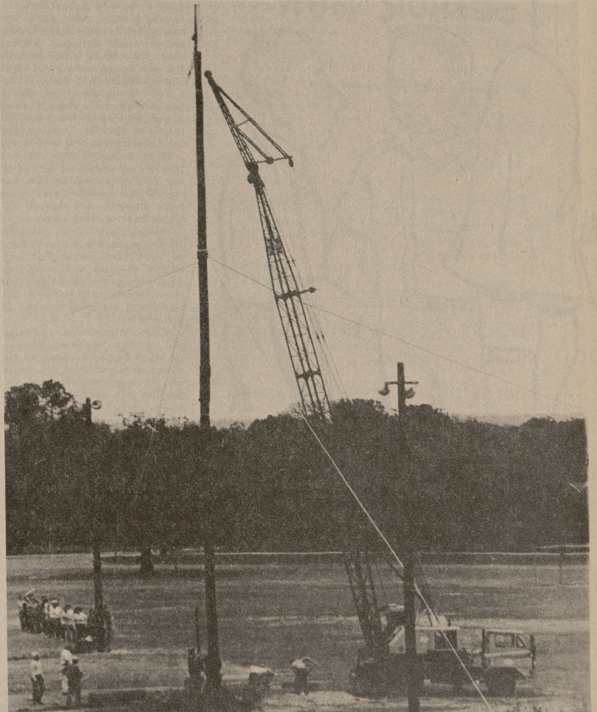
IT'S UP! And so work can begin on the 1972 bonfire for the A&M-Texas game. The 90-foot pole was put up Thursday in two 60-foot sections with 15 feet buried underground and 15 feet used for splicing. Juniors and seniors will be able to do preliminary woodcutting next week. (Photo by Robert Franklin)
