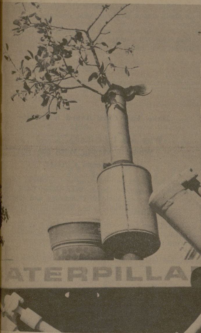
MAY BE AN ECOLOGY STATEMENT or just terrible driving but it is an oak branch sticking out of a bulldozer's exhaust stack. Poor driving must not be discounted because the dozer is at the construction site across from The Exchange Store, location of at least two amusing bogging-down incidents in past days. (Photo by Robert Williams)
