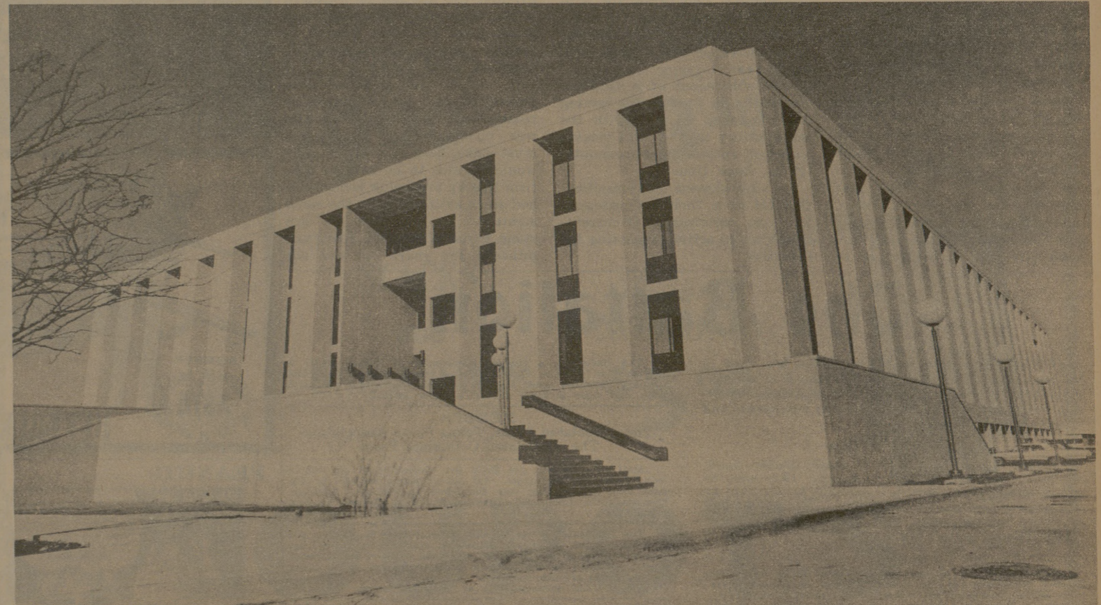
MONDAY IS MOVING DAY as several engineering departments transfer to the new $10 million Engineering Center located on the north side of the campus. The move
