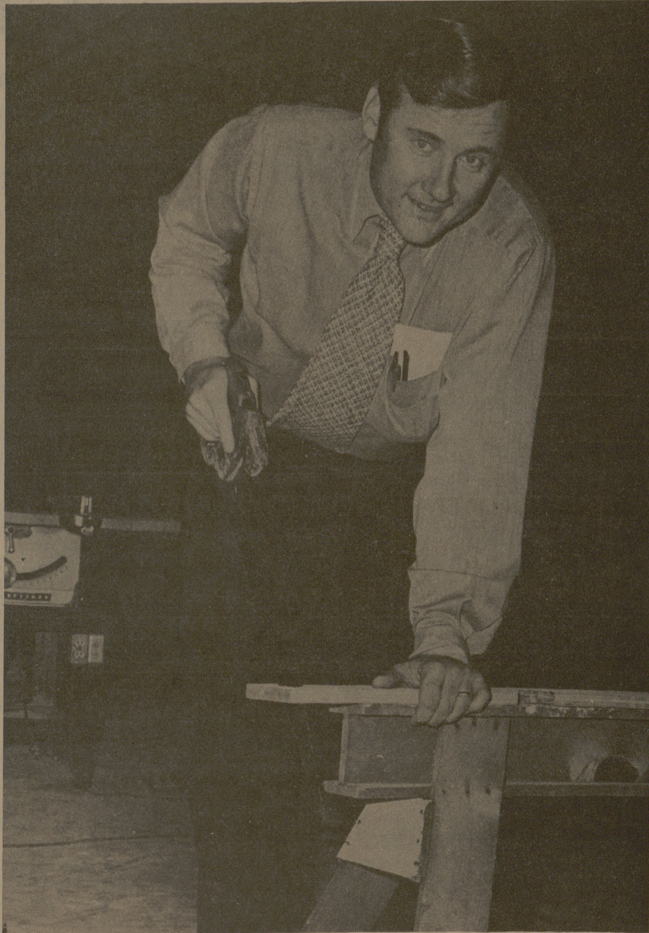
Rusty Rush, Co-Owner of the Country Squire, Helps With the Construction During The Remodeling.
