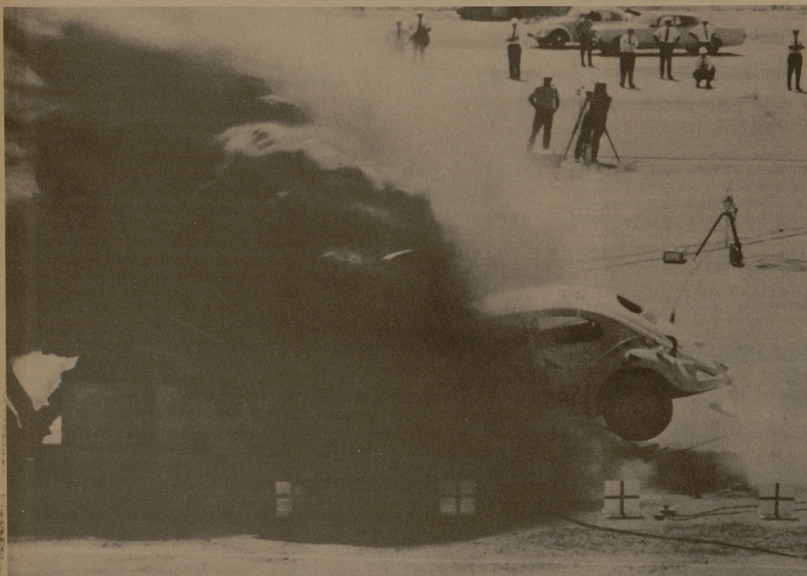
A SMALL CAR TRAVELING at 60 miles an hour and controlled by radio hits tubs of sand, escaping serious damage in a test by engineers for the California Division of Highways. The engineers are using the tubs of sand plus water-filled tubes and empty steel barrels to prevent cars from slamming into such fixed objects as bridge railings and signposts along freeways. (AP Wirephoto)
