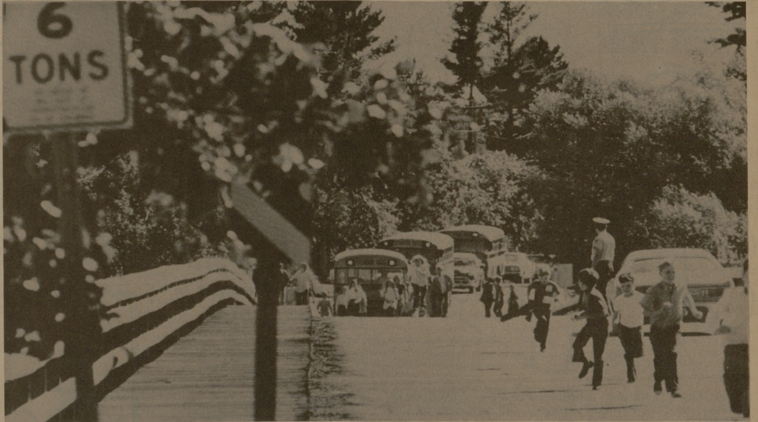
SINCE THE SCHOOL YEAR OPENED Wednesday, 140 youngsters disembark from three buses twice each day to cross this bridge near Chetek, Wis. Highway officials lowered the bridge's weight limit to six tons this summer.
