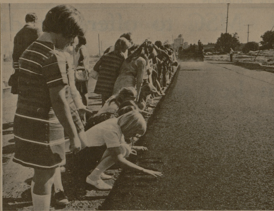
CHILDREN TAKE A LOOK at and get the feel of a city street in Fullerton, Cal., which is the first in the nation made with a new paving material composed of more than a million used glass bottles and called glasphalt. The road is in a relatively remote area and is only 600 feet long. It is made of almost the same materials used for asphalt paving, with glass substituted for gravel and stone. (AP Wirephoto)
