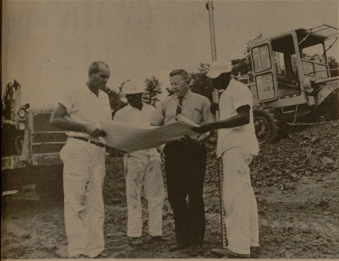
TWENTY-ONE INMATES OF THE ELLIS PRISON unit near Huntsville are enrolled in the heavy equipment school here at A&M. They are currently building a 13 mile levee on the unit under the direction of A&M and planning by the Army Corps of Engineers. Pictured are, Al Jones, chief instructor of the school, and (from left) James Koonce, Hickey McCook and Thomas Oliver, inmates.
