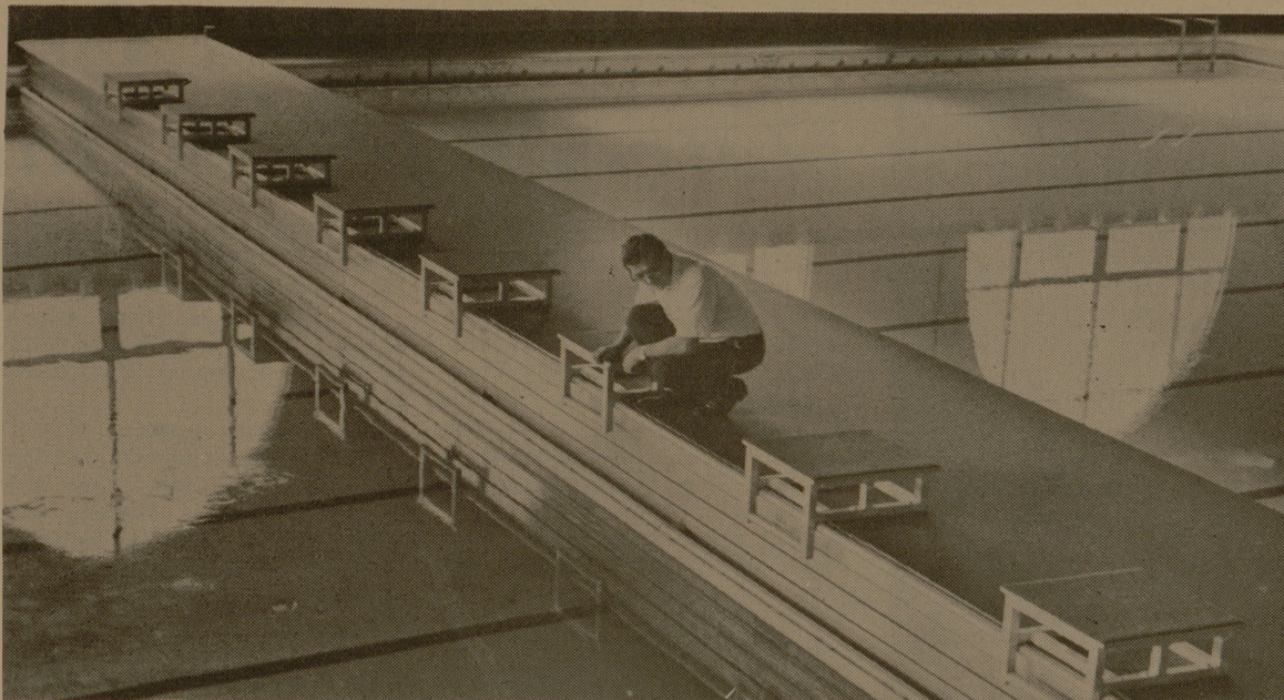
A carpeted bulkhead shortens the P. L. Downs pool to championship length.
