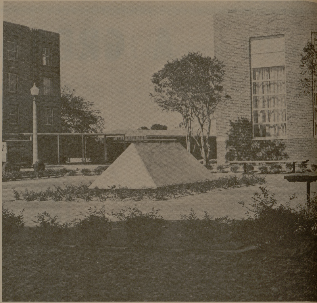
MEMORIAL ALMOST FINISHED
