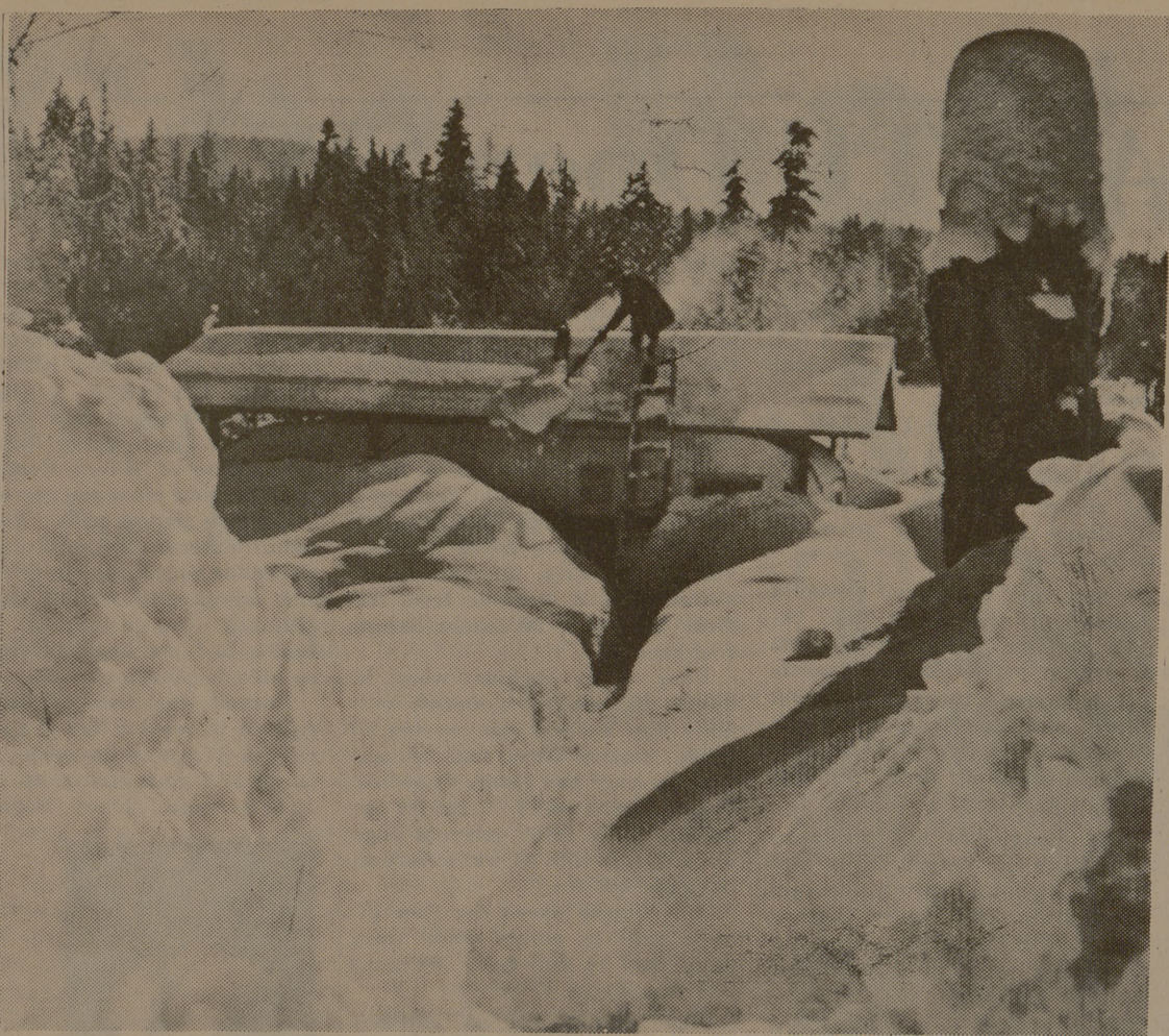
Roof shoveling has been common around Spokane, Wash., this winter as residents work to keep buildings from collapsing under the weight of 42 inches of snow. Pacific Northwest people are referring to this as the year of the "supersnow," since tons of the stuff has buried most of this corner of the nation. (AP Wirephoto)
