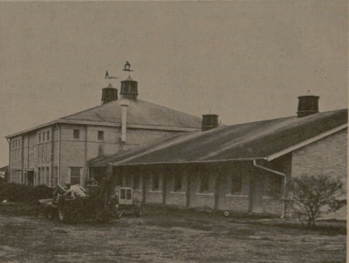
PROGRESS CONTINUES Another of A&M's famous landmarks—Garrigan's horse barn—has fallen victim to the rapid changing university which has long since entered the space age. The barn, built in 1933 for $25,000, is undergoing renovation to the tune of $100,000 to house the fast-growing Recreation and Parks Department.
